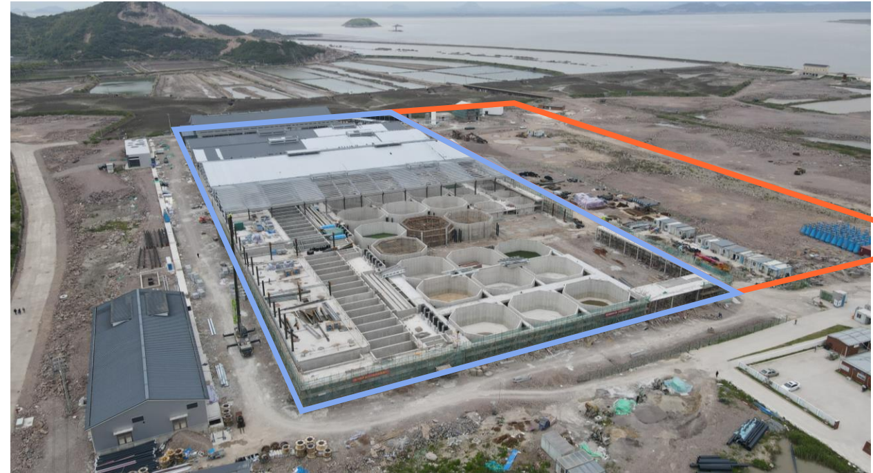
Construction site April 2023
