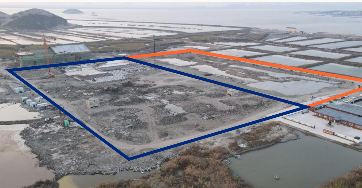
Construction site early December 2021
