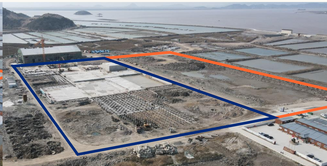
Construction site early March 2022
